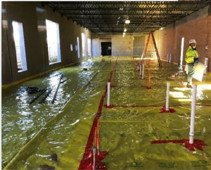
Underground plumbing and prep work for the concrete floors
