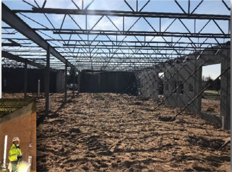
Structural steel, roof joist, metal decking
